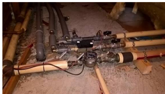
Energimåler i skunk for 1.sal. Varmeinstallation mangler isolering.
